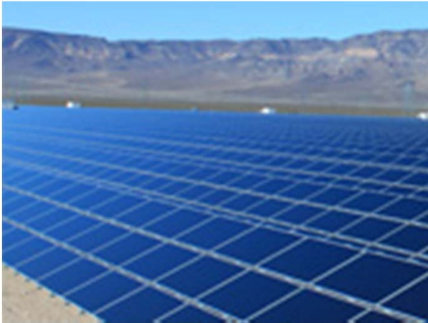
Copper mountain PV plant, Boulder City
