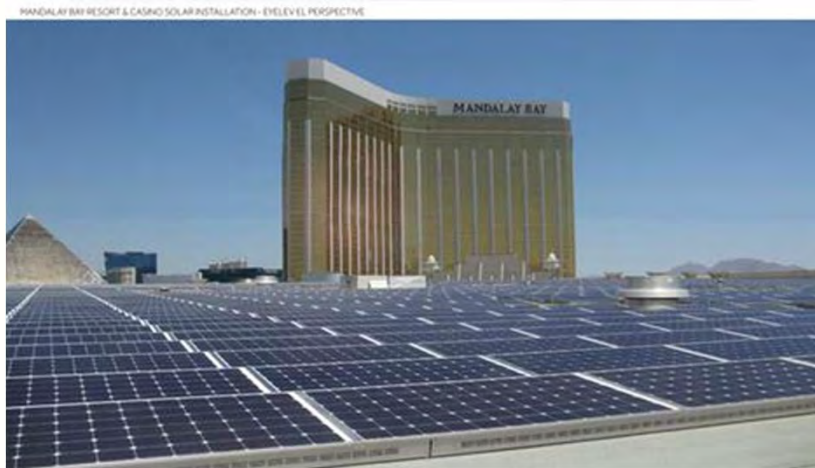
Mandalay Bay Convention Center Solar Project – Las Vegas “not constructed yet”
