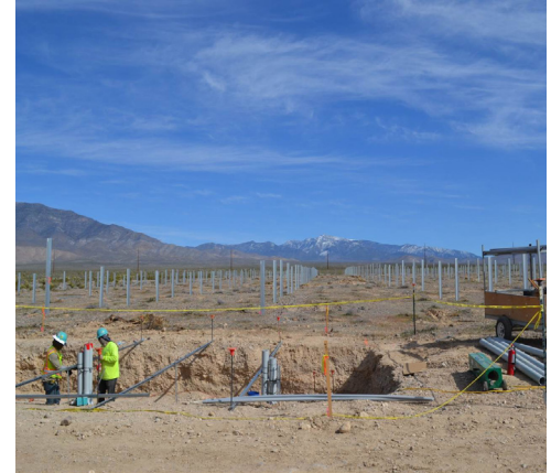
VEA Community Solar Project Construction --VEA Photo
